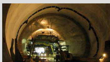
Izolace s chráničkami pro kabely. Membrane waterproofing with the cable protectors.
