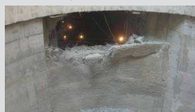
Prorážka tunelu do šachty. Tunnel breakthrough into the shaft.
