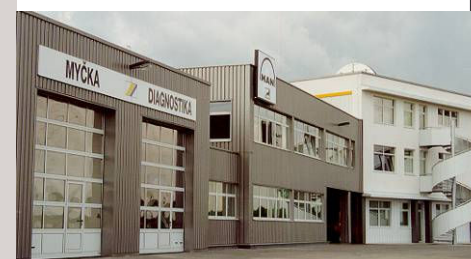
■ MAN – Průhonice – service and administrative centre
