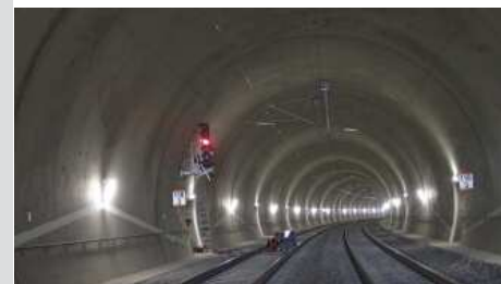
■ Railway tunnel Olbramovice, line Prague/Linz
